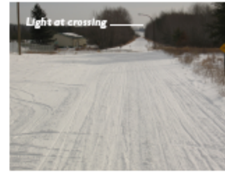
Along with proper signage, a light is added at this trail crossing to improve safety. The flatness and straightness of this roll conversion reduced the visual cues associated with identifying this intersection, warranting the addition of the light.
