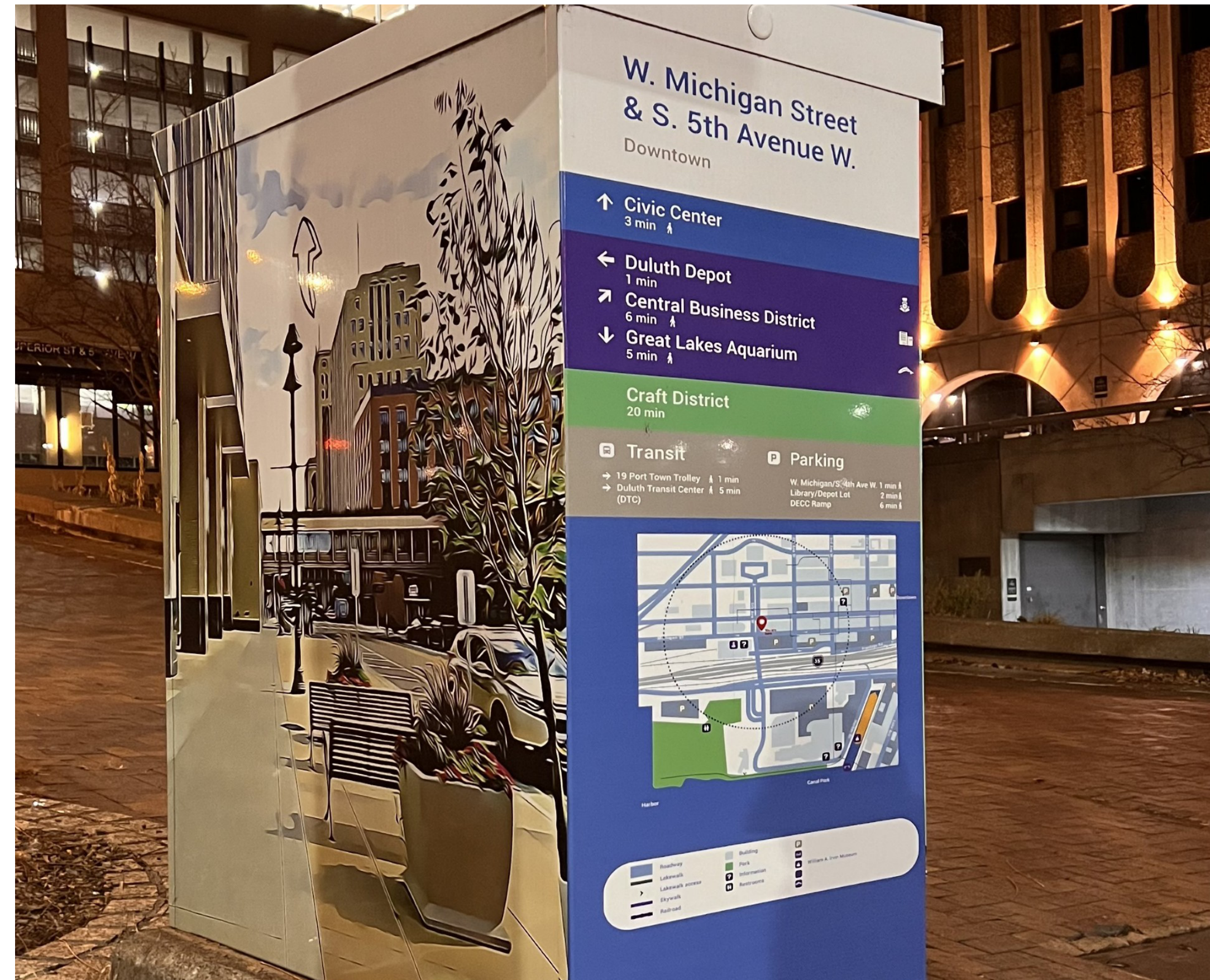
A utility box at the corner of 5th Avenue West and West Michigan Street, exhibiting public art and wayfinding signage.
