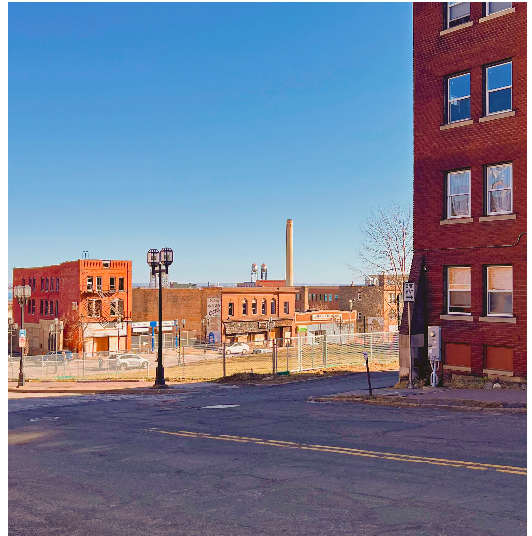
The former Pastoret Terrace (also known as the Kozy) building, at the northeast corner of West 1st Street and 2nd Avenue East, is a redevelopment site owned by DEDA.
