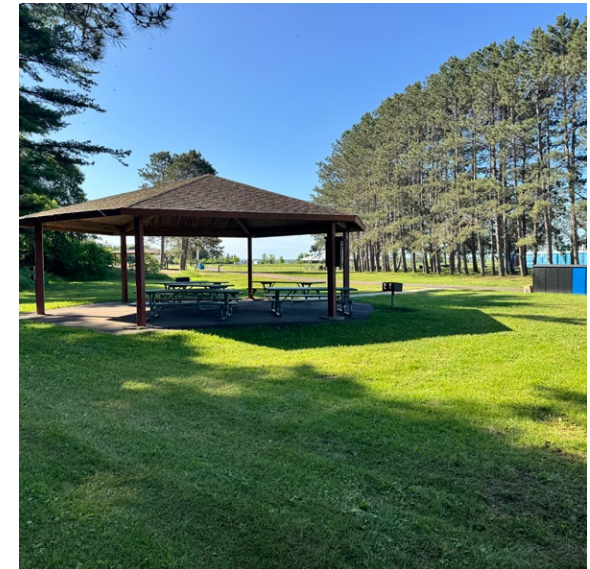
Figure 02.24 Existing picnic shelter
