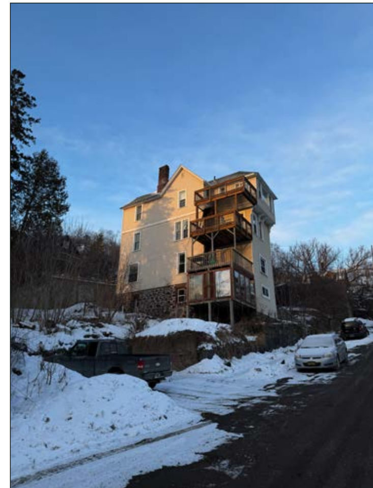
Existing View from SW
