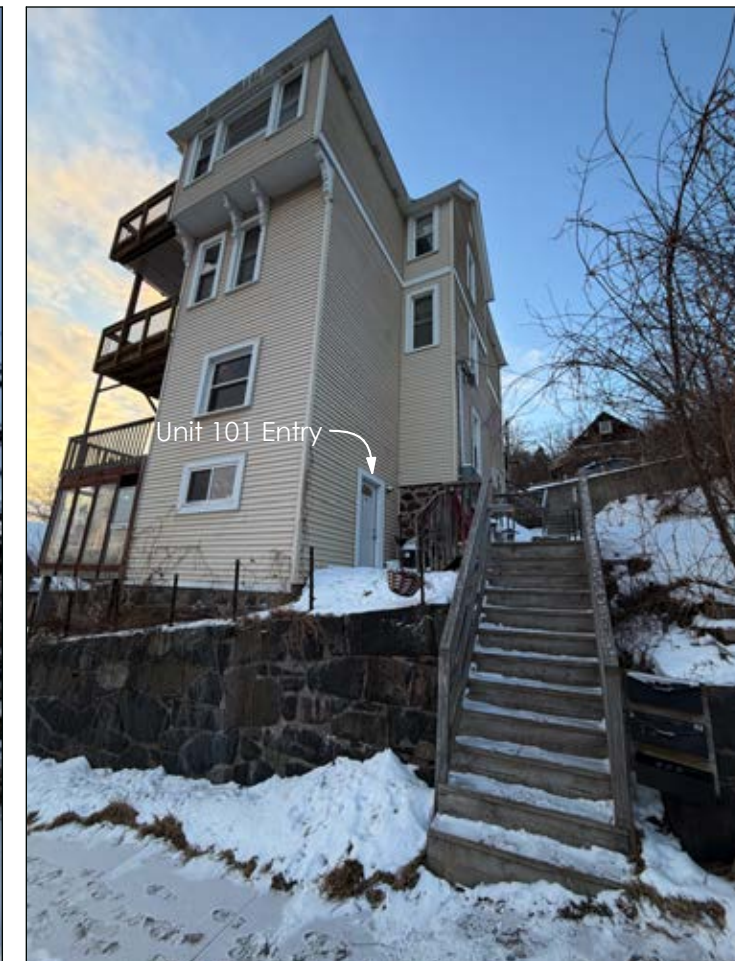
Existing View from SE
