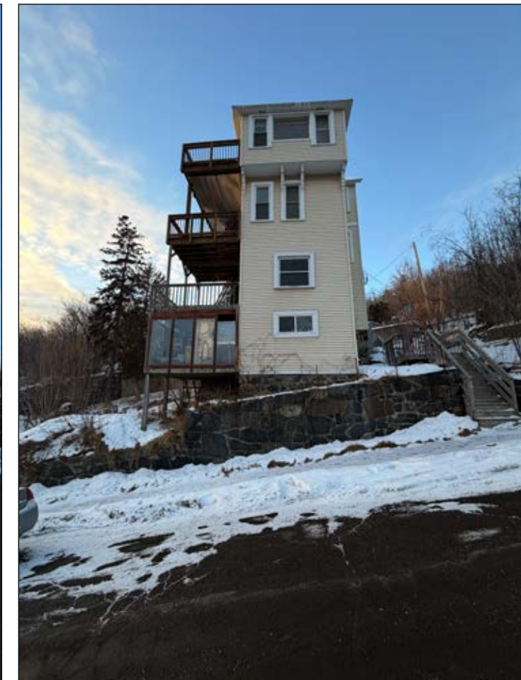
Existing View from South
