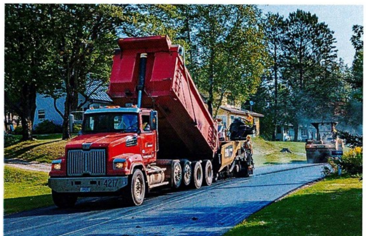
Lawn Street paving, September 2024.
