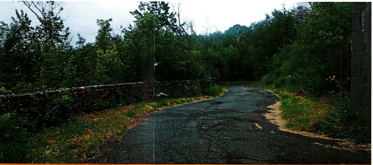
Full-depth reclamation, ditching, and storm sewer improvements can help drain and strengthen grade on Lincoln Park Drive.
