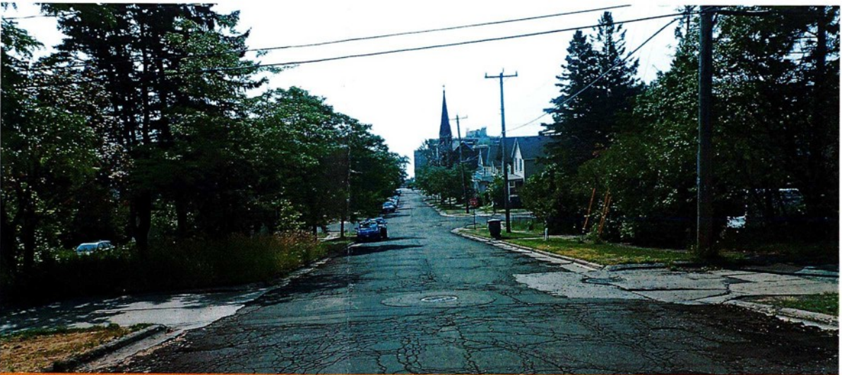
Drainage improvements would include repair or replacement of deteriorated catch basin structures.
