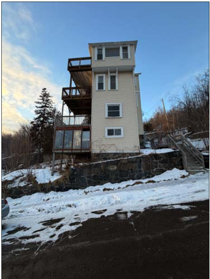
Existing View from South
