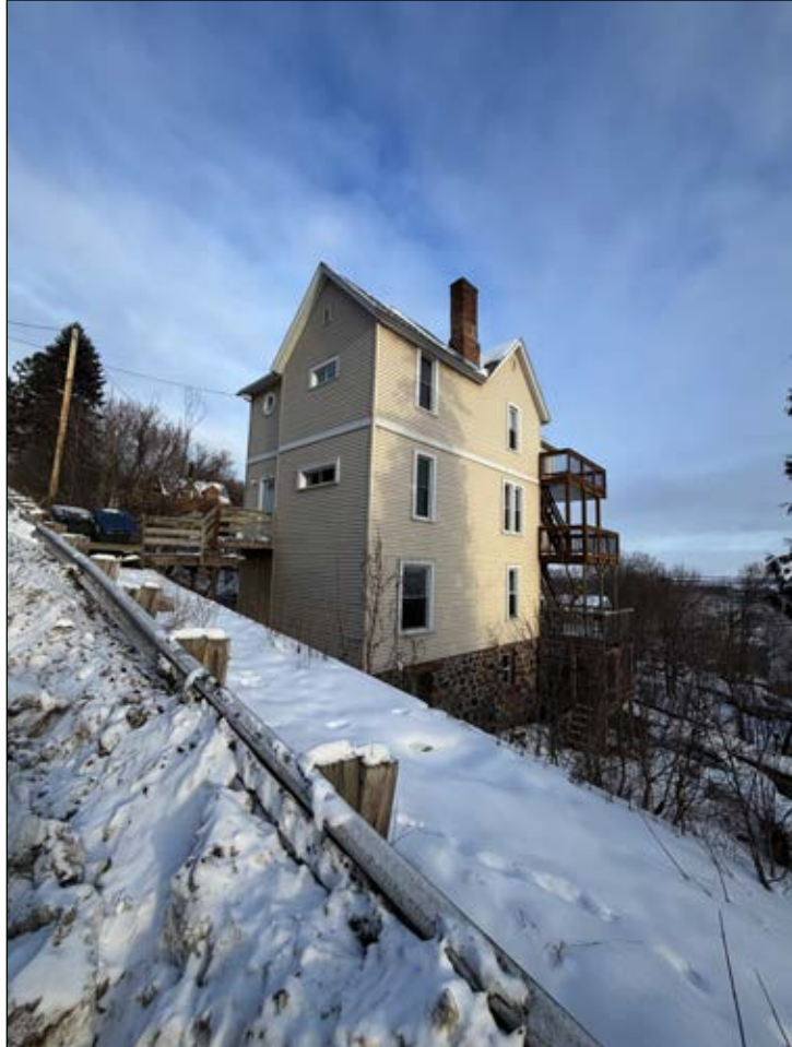
Existing View from NW
